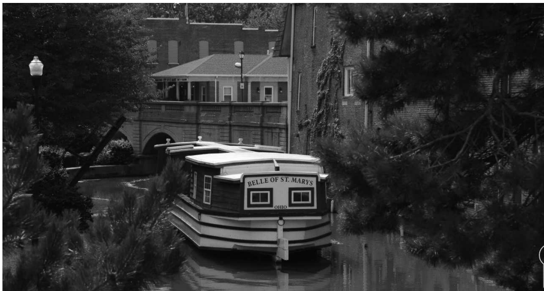
Figure 31: The Miami-Erie Canal as it flows through historic St. Marys showing the red brick buildings that sustained structural earthquake damage from the 1986 4.5 earthquake. Source: https://seemore.org/play/lake-life/the-aqua-life-at-grand-lake/
